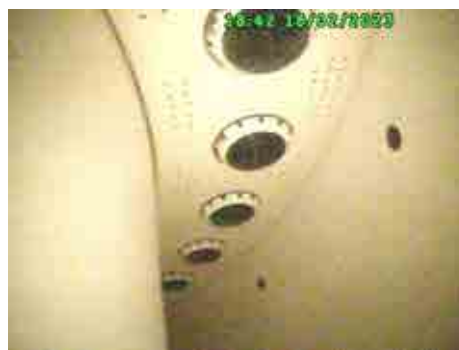
Front panel with burners from burner#22.
