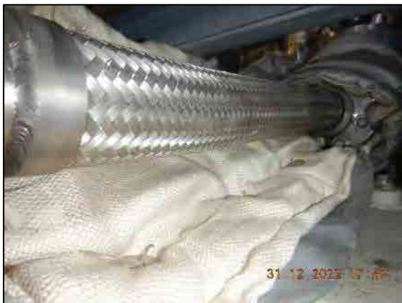
Example of gas fuel supply flexible hose overall condition.
