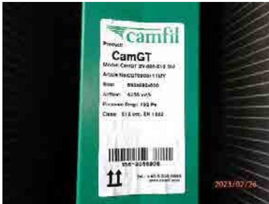
Installed fine filter CamGT 3V-600-E12 Std.
