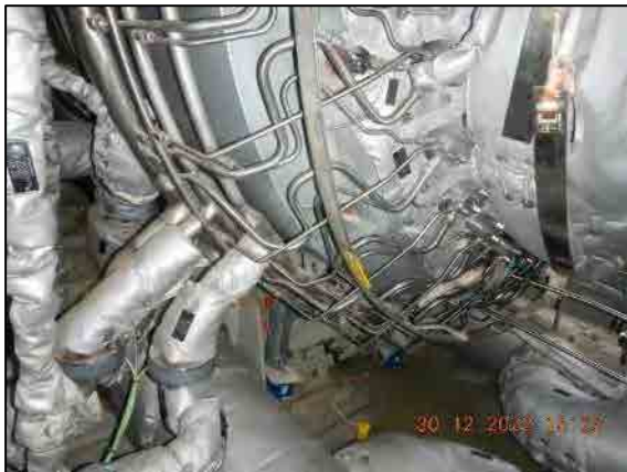
Gas fuel supply manifold connection area.
