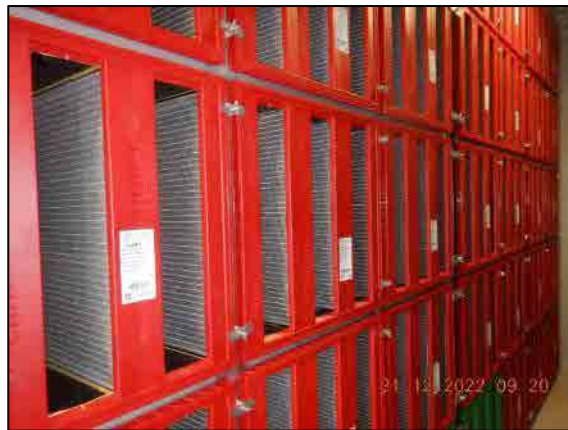
Example of fine filter element contamination.
