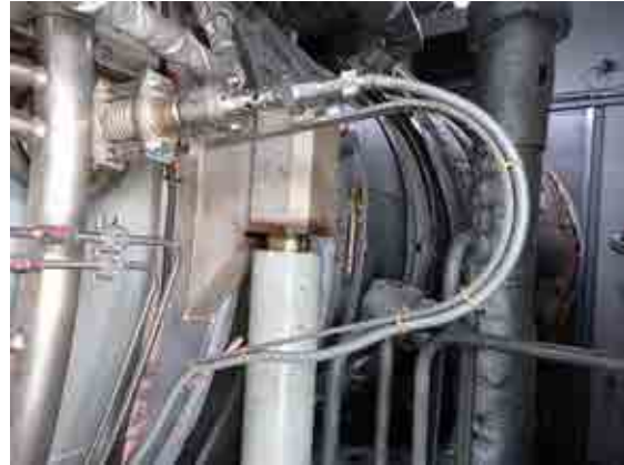
Flame detector on the right-side overall condition.
