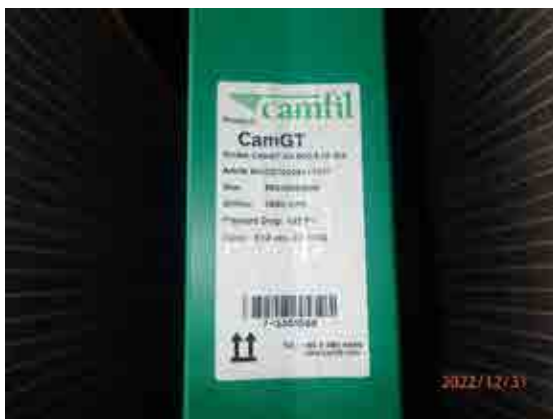
Installed fine filter CamGT 3V-600-E12 Std.
