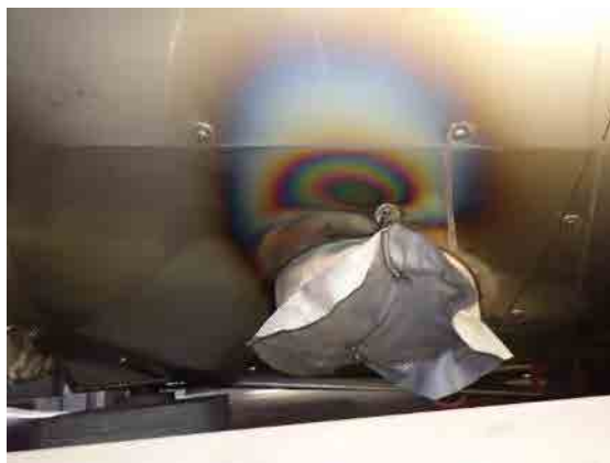
Hot air leaked sign right side
