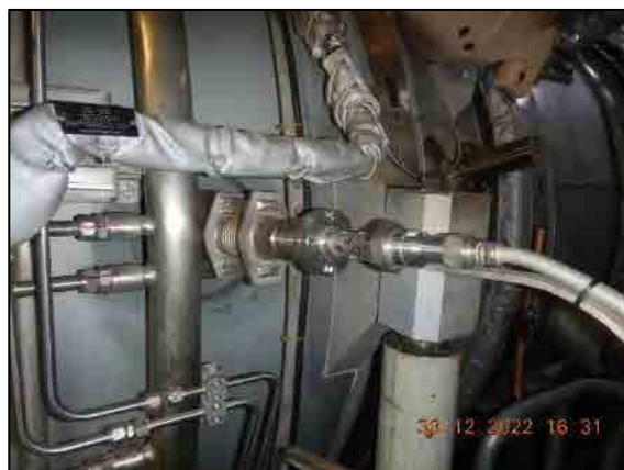
Flame detector on the right-side overall condition.
