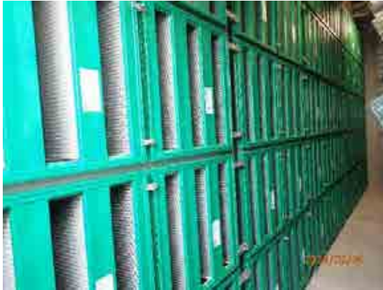
E12 fine filter overall condition.
