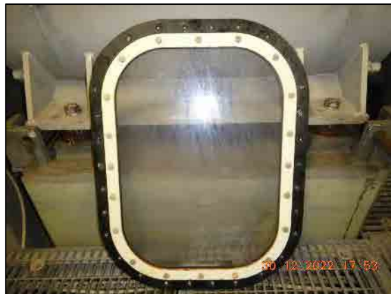
Sight glasses rubber seal condition.
