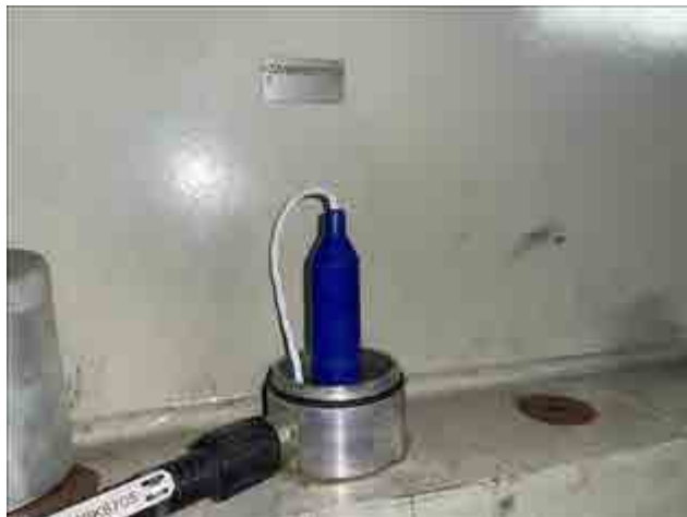
9 VB sensor was cleaned and still tightened.
