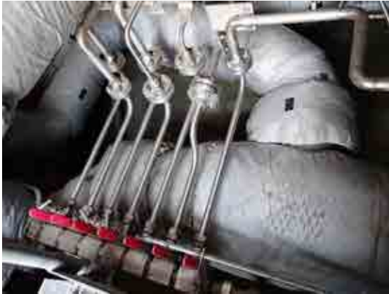
Drain valves overall condition.
