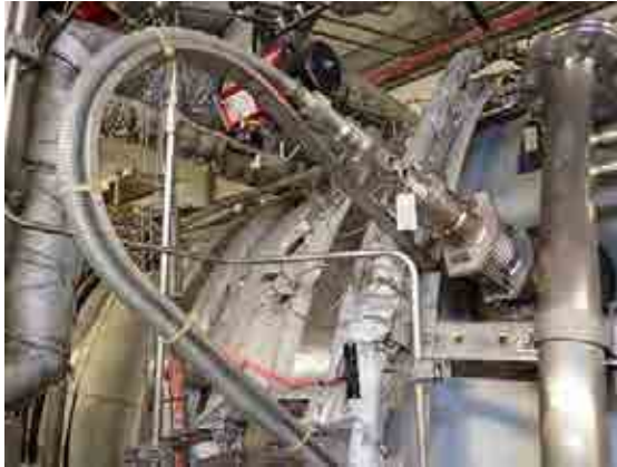
Flame detector on the left-side overall condition.
