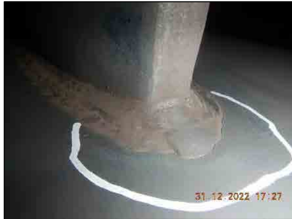
Example crack found at this area.
