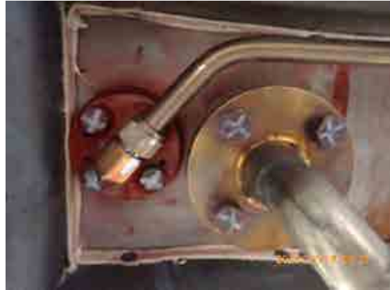
CC casing drain port as found condition (No leakage)
