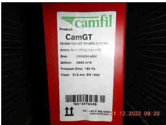
Installed fine filters are CamGT 3V-600-E12 Std.
