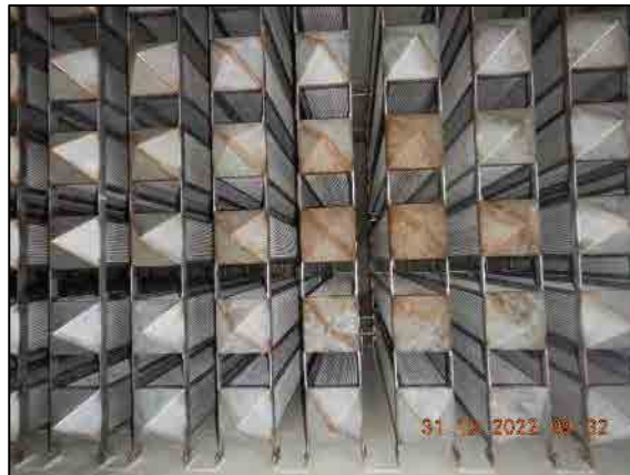
Example of surface corrosion found on silencer unit.
