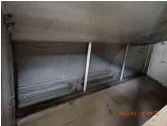
Clean air exit to enclosure ventilation unit.
