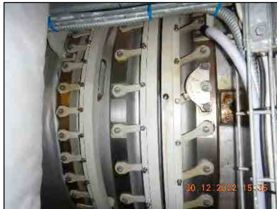
GV arms and lever mechanism on left side.
