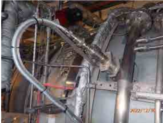
Flame detector on the left-side overall condition.
