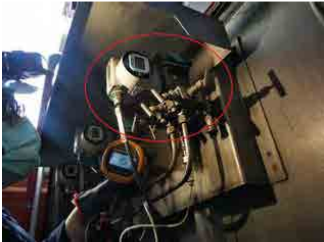
51 SAG10CP010 pressure transmitter deviation
