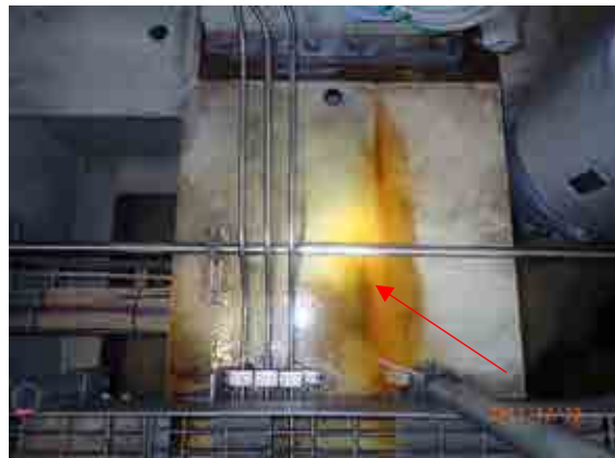
Found lube oil on foundation under right junction box.
