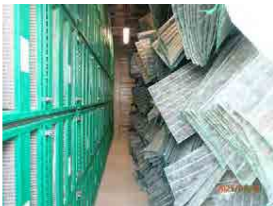
Inside intake filter housing overall condition.
