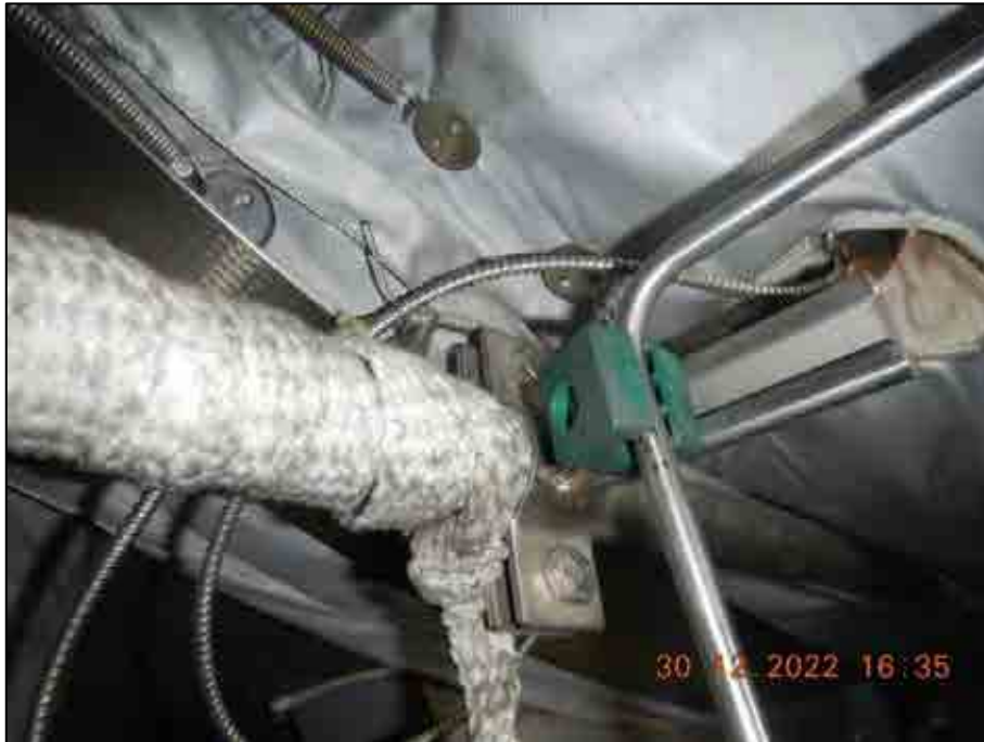
Bracket locking jacking oil pipes to bearing 2 found broken.
