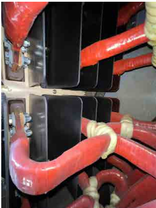
6 Stator winding connention
