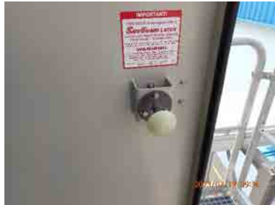
Intake door push open mechanism good condition.
