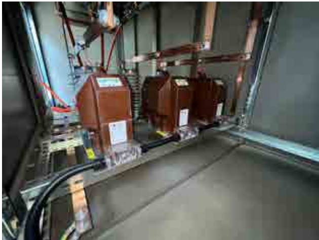
12 Voltage transformer
