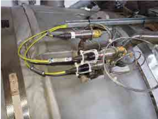
Vibration sensor to bearing 2 overall conditions.
