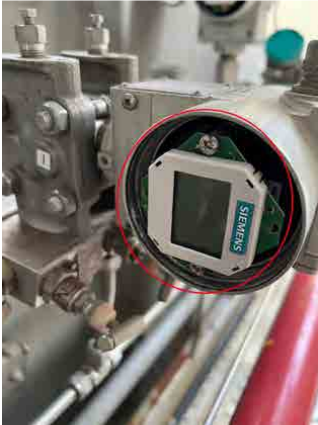
4 MBA10CP040 pressure transmitter display malfunction
