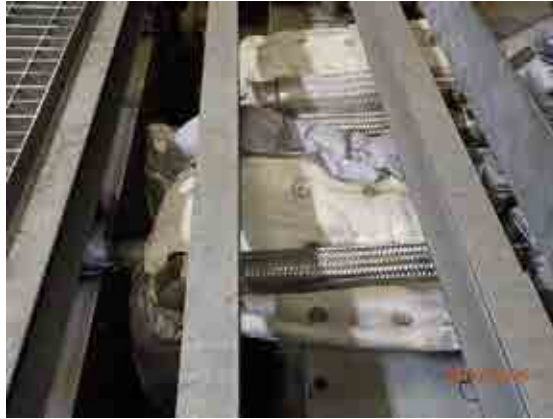
Gas flexible hoses condition
