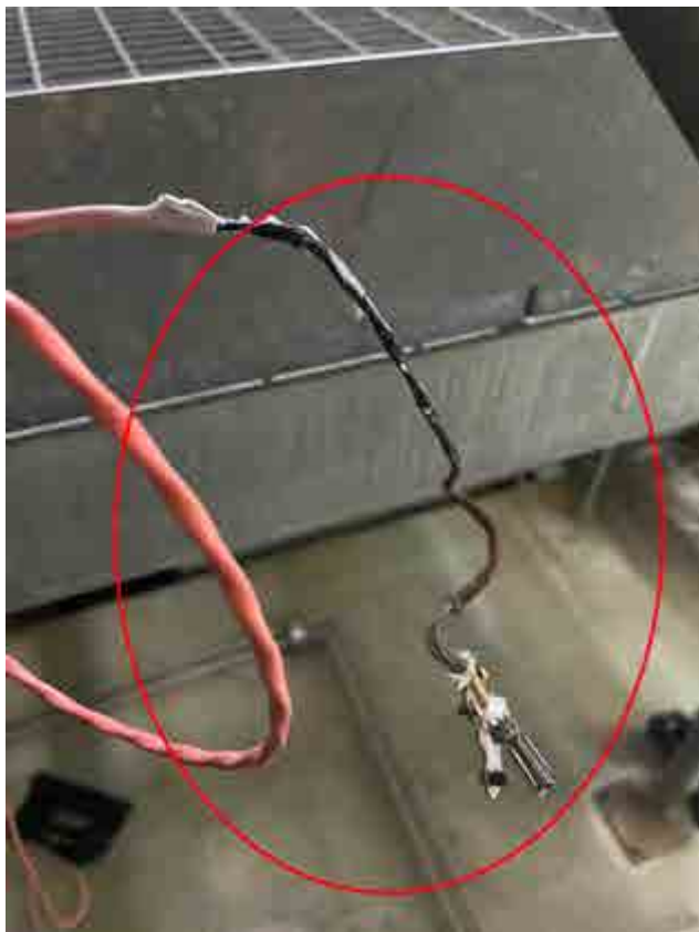
11 MBA10CT050 Cable damaged
