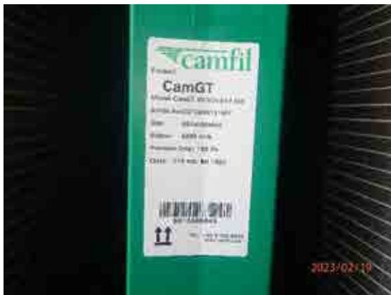
Installed fine filter CamGT 3V-600-E12 Std.
