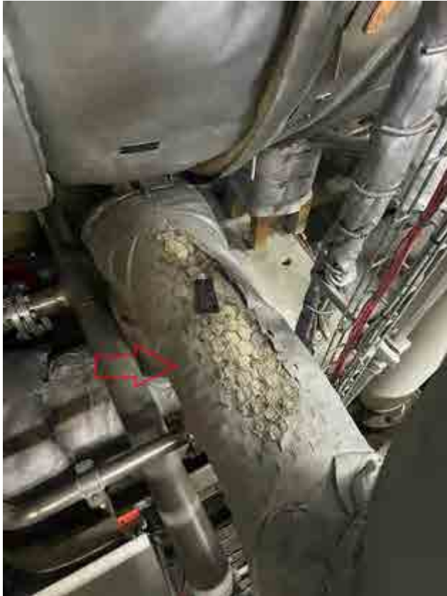
1 Damaged insulation blanket (2)
