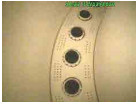
Front panel with burners from burner#1.
