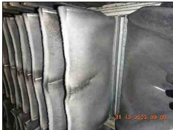
Example of contamination condition on filter element.
