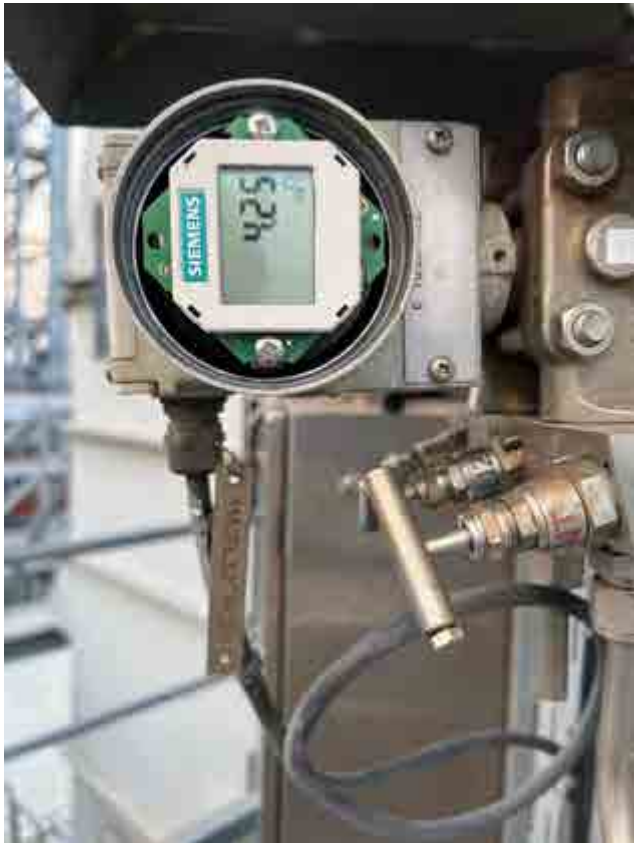
17 MBL30CP030 pressure transmitter deviation
