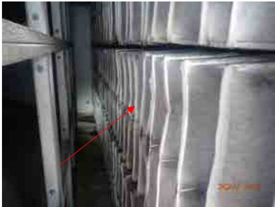
Ventilation filter elements fouling condition.
