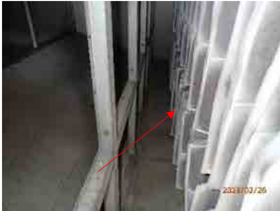
Ventilation filter elements fouling condition.
