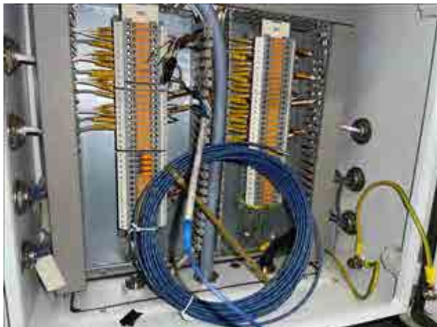
8 Temporary RTD has been connected.
