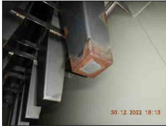
Example of surface corrosion found on some of the silencer.
