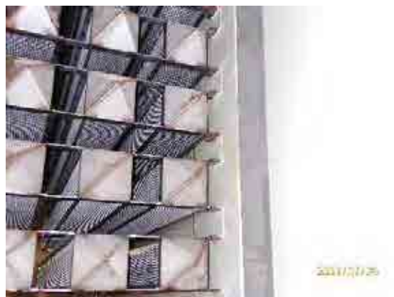
Close up on silencer unit flat bars weld joint condition.
