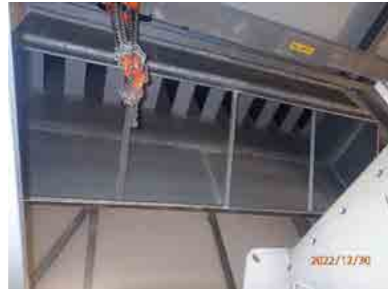
Ventilation silencer exit to enclosure.
