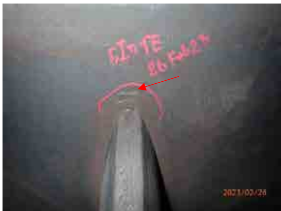
Example of crack at front support struts.
