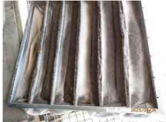
Ventilation filter elements fouling condition.
