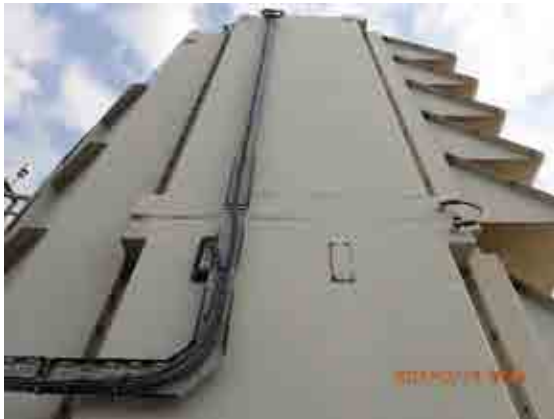
Algae cover inlet filter housing condition.
