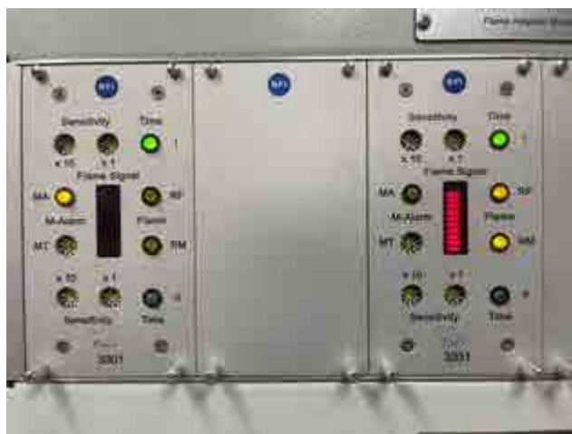
5 Flame detector function check
