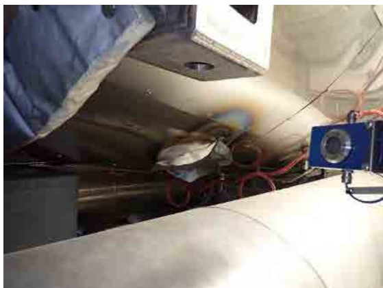
Hot air leaked sign bottom side
