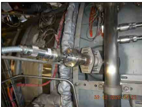
Flame detector on the left side overall condition.
