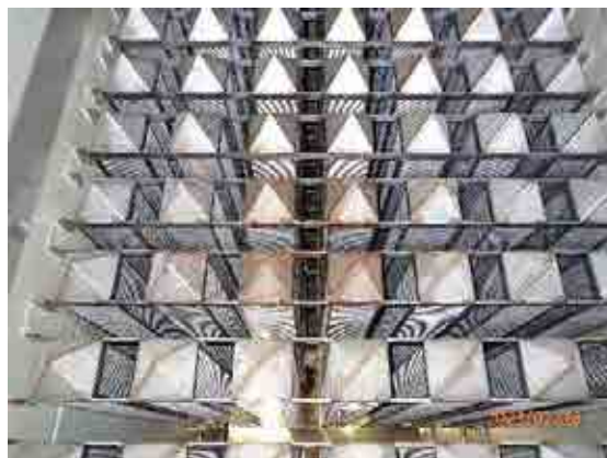
Silencer unit intake side close up condition.
