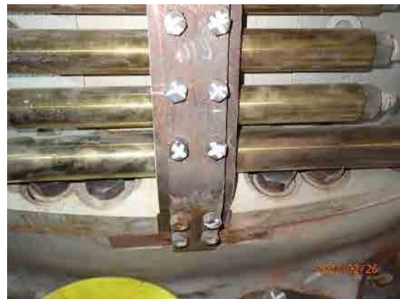
Bottom side guide collar as found condition.
