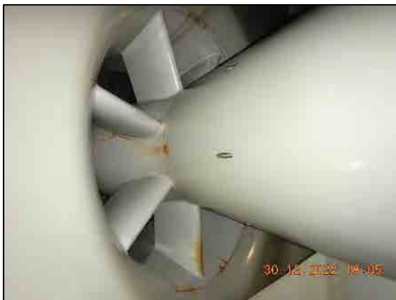
Left side dirty water trace condition.
