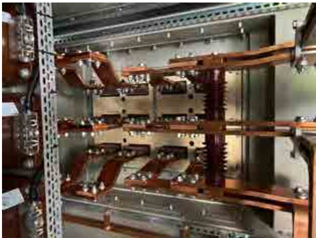
11 Line and neutral connection
