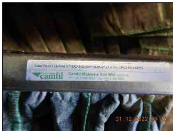
Installed pre-filter element were CamFlo GT Hybrid X7.
