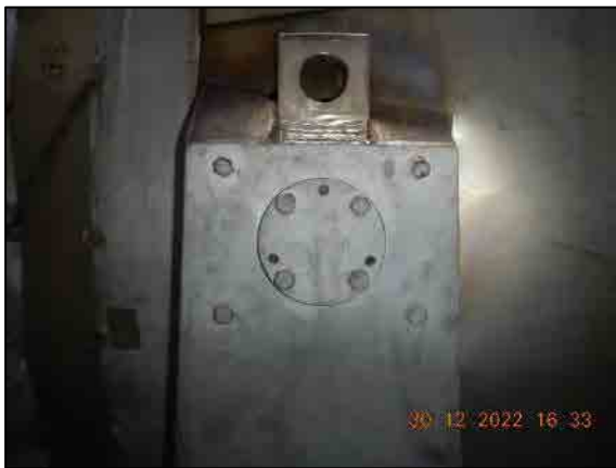
Right side exhaust diffuser support condition.
