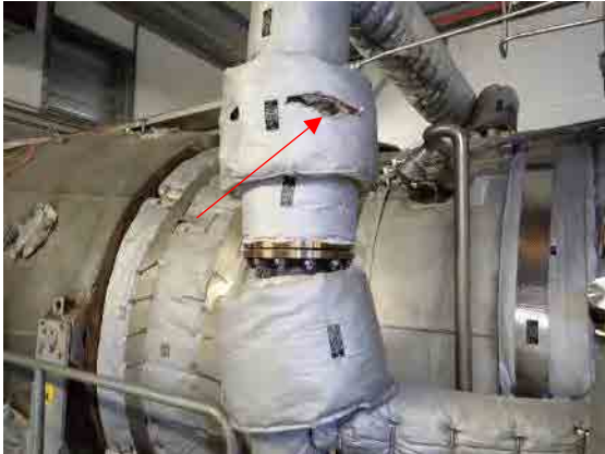
Condition of insulation on cooling and sealing air pipe. Condition of insulation on cooling and sealing air pipe.
