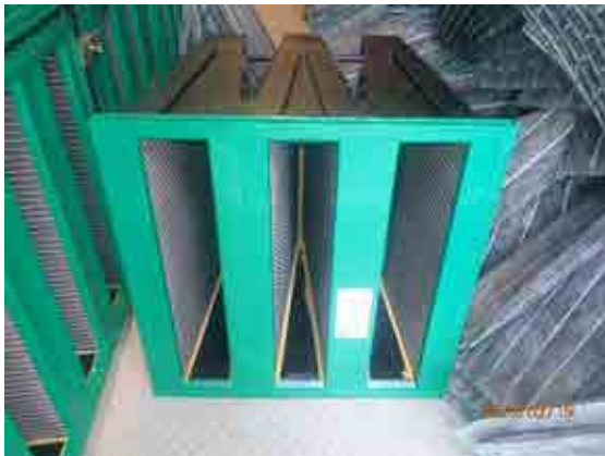
Fine filter as found condition.
