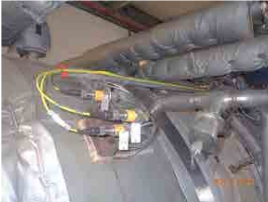
Vibration sensor to bearing 2 overall conditions.
