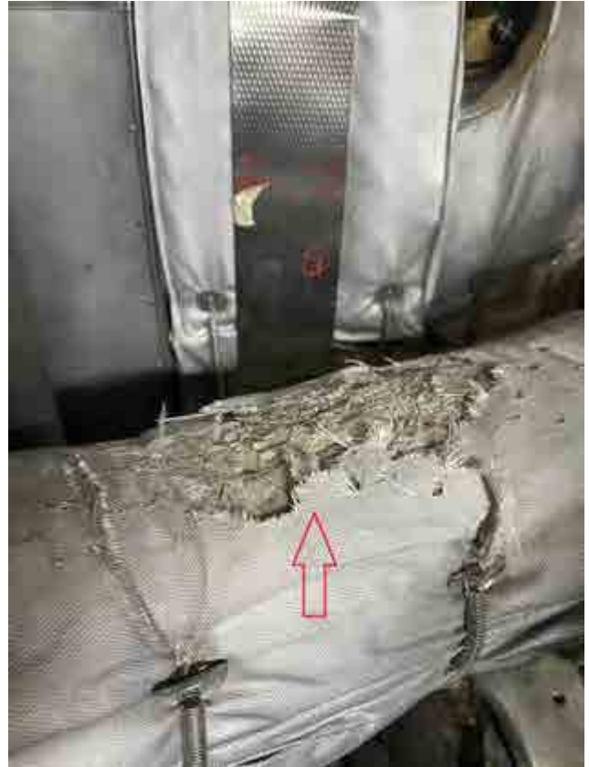
1 Damaged insulation blanket
