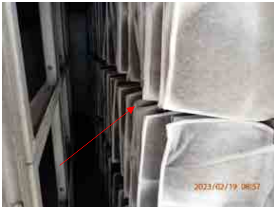
Ventilation filter elements fouling condition.
