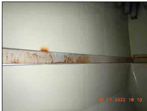
Example of corrosion found at this area.
