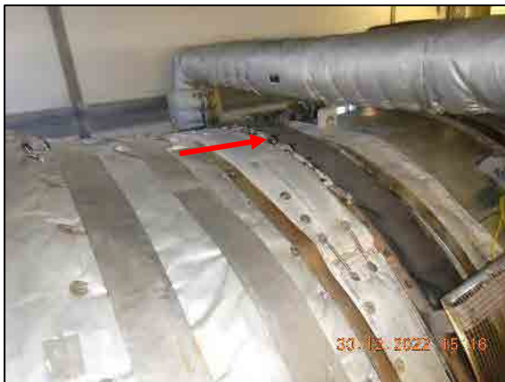
Flexible part soft skin damaged notice.
